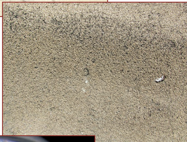
Figure 37. A closer view of granule loss of localized granule loss occurring as a result of contaminants from bird droppings.
