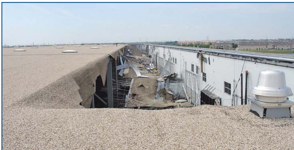
Figure 1 – A typical drainage-related collapse of a low-slope roof. Photo by Stephen Patterson.
