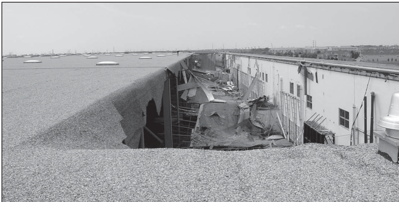
Figure 4 – An example of a typical roof collapse caused by inadequate roof drainage.
