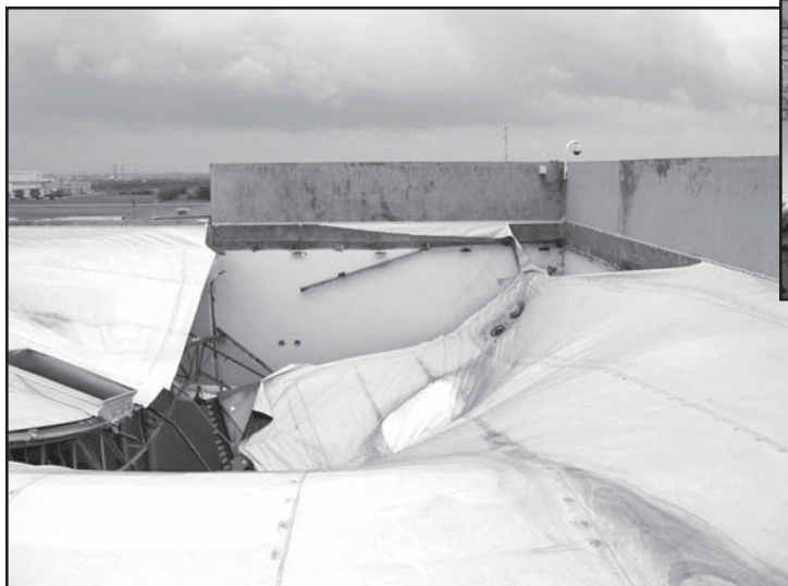
Figure 9 – Photographs of the collapse of a low-slope roof in Fort Worth, TX, due to the combination of wind and rain loads. (a) Left: Photograph showing the collapse from above the roof. (b) Above: Photograph showing the collapse from the inside.
