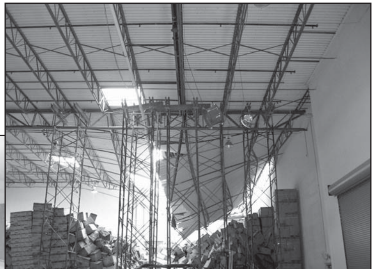
Figure 9 – Photographs of the collapse of a low-slope roof in Fort Worth, TX, due to the combination of wind and rain loads. (a) Left: Photograph showing the collapse from above the roof. (b) Above: Photograph showing the collapse from the inside.
